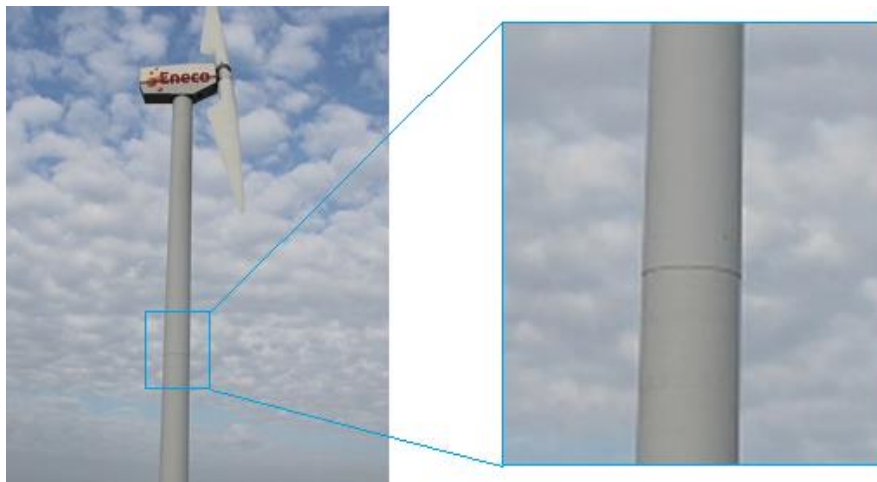
Figure 5 - Duinvogel slip-joint in-situ
