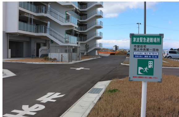
Indication evacuation building
