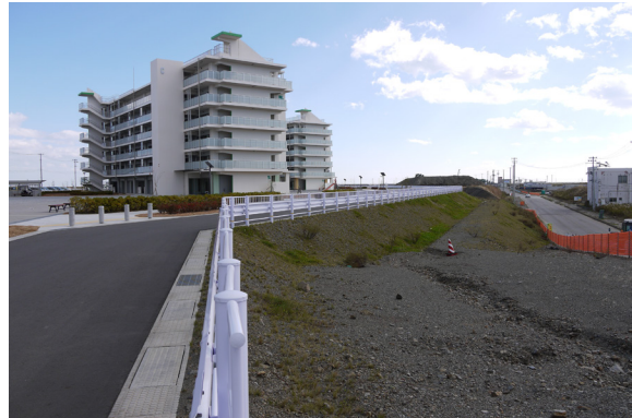
Reconstruction on elevated landfill
