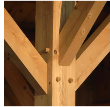
Figure 37 Sawn timber assembly
