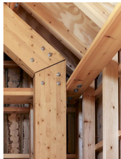
Figure 33 Dowelled connection with slotted-in plate
