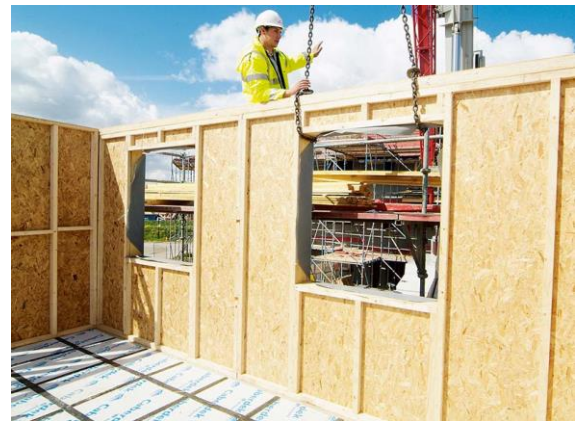
Figure 15 Timber house under construction
