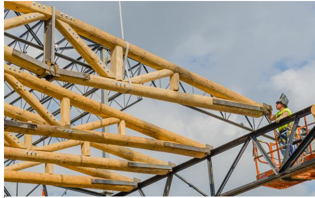
Figure 35 Round wood trusses
