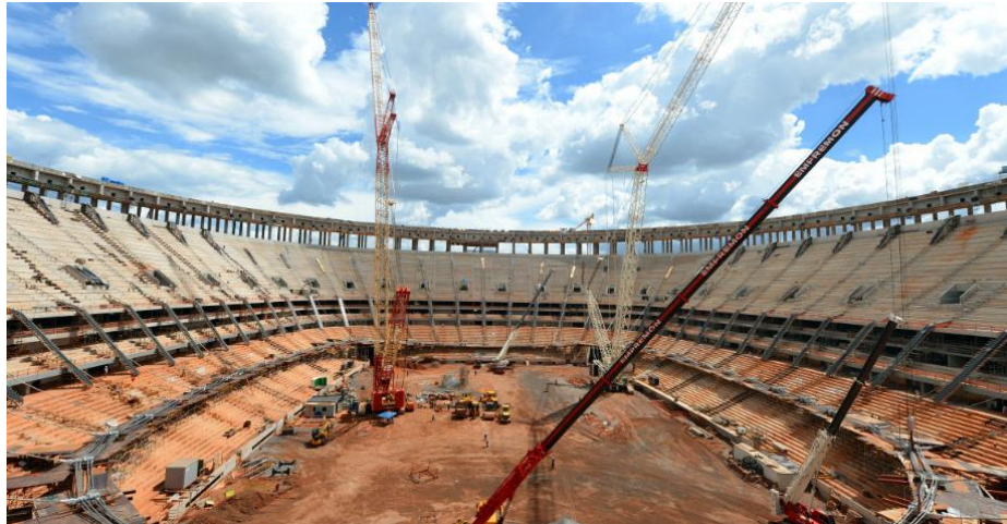
Figure 6 World cup stadium under construction
