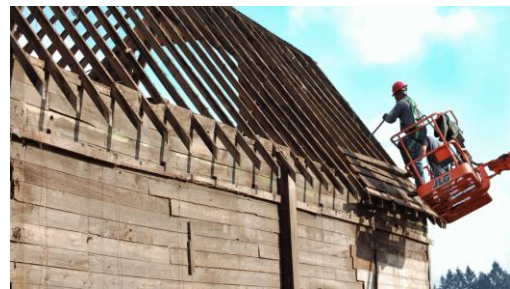
Figure 18 Workers dismantling a timber roof
