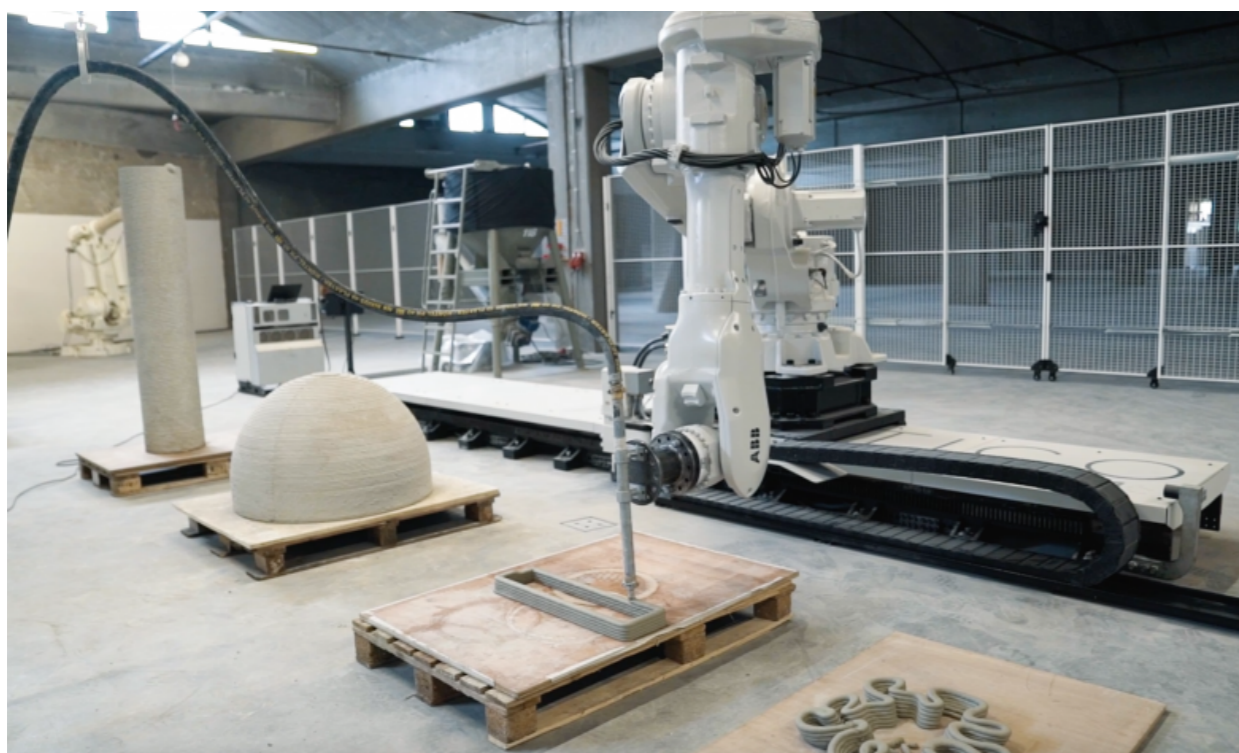
image / figure 2: 3D Printing with concrete
