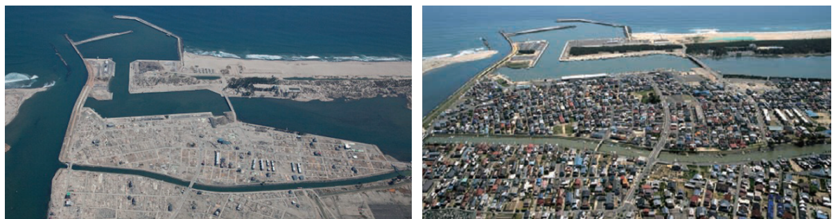
Figure 4.3: Before and after the tsunamis in Yuriage district (Natori city)
