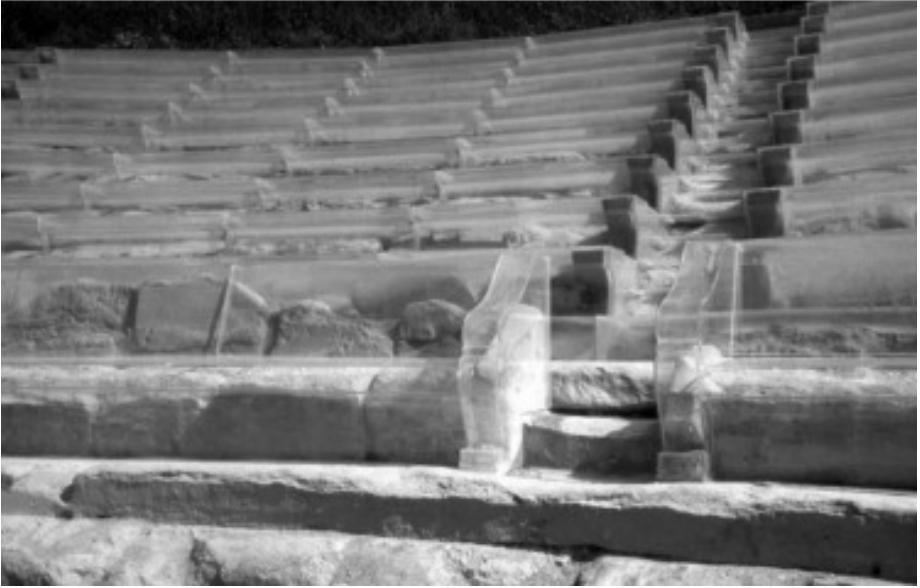
Figure 5. Restoration of the Theater of Heraclea Minoa (Sicily) by F. Minissi. Plexiglas is used to revive the original shape of the seats (Vivio 2014).
