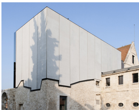
Figure 2a. The new façade of Louvoiers Music School (France) was restored using prefabricated reinforced concrete panels, cut out to follow the surface of the historic masonry showing the distinct boundary between the old and the new (Dent 2012).
