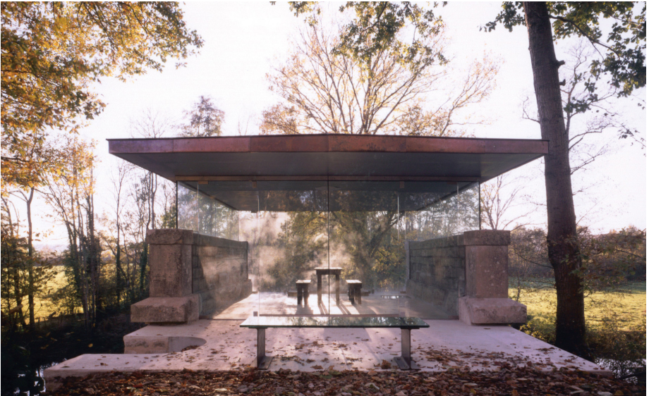
Figure 6. The temple de l' amour II in Burgundy (France) uses glass plates of minimal thickness to carry the compressive loads of the roof creating a full panorama (Kraaijvanger 2018).
