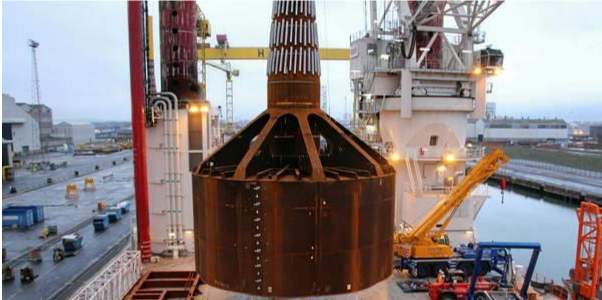
Figure 10 – Mono-bucket foundation (source: Universal Foundations)
