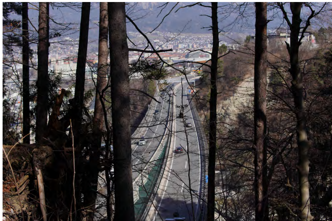
88 | Highway through Innsbruck
