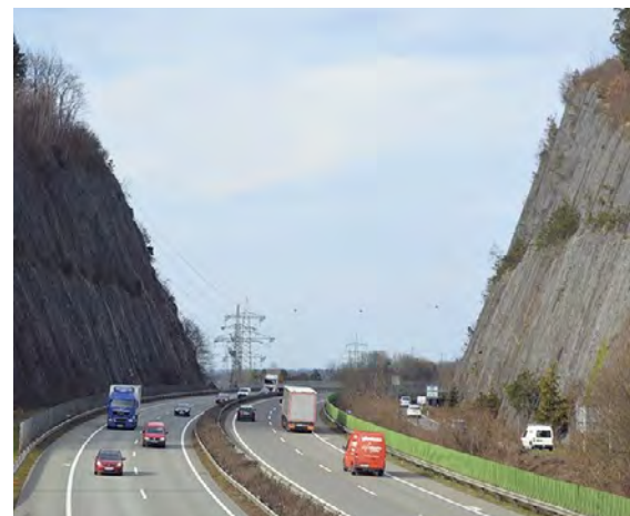
62 | Blown up part of the Udelberg, to make way for the A14 highway (Autor unknown)
