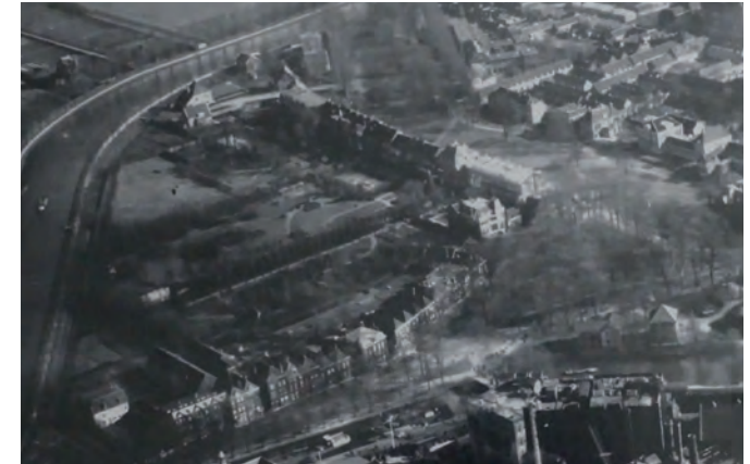
Figure. 2.58. - Aerial photograph of Waller and Tutein Nolthenius garden, circa 1910 - Image from Archives Teun van Staveren
