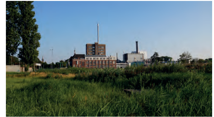
Figure 1.3. - Former Calvé terrain in an overgrown state
