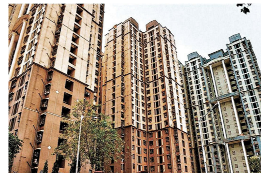
Fig.5. CIDCO mass housing scheme
