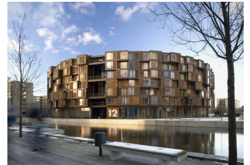
Tietgen Dormitory by Lundgaard & Tranberg
