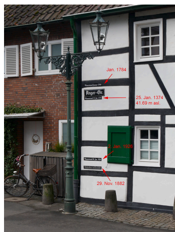
Fig. 2. Water level related to the 1374 flood event at Düsseldorf-Urdenbach (Photo: Jürgen Herget).
