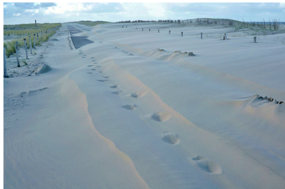
Figure 1.2: Buried bicycle/footpath in the Hondsbossche Dunes as a result of high velocity onshore directed winds. Hondsbossche dunes, 3-2-2016 [Fortuijn and Van Egmond, 2018]
