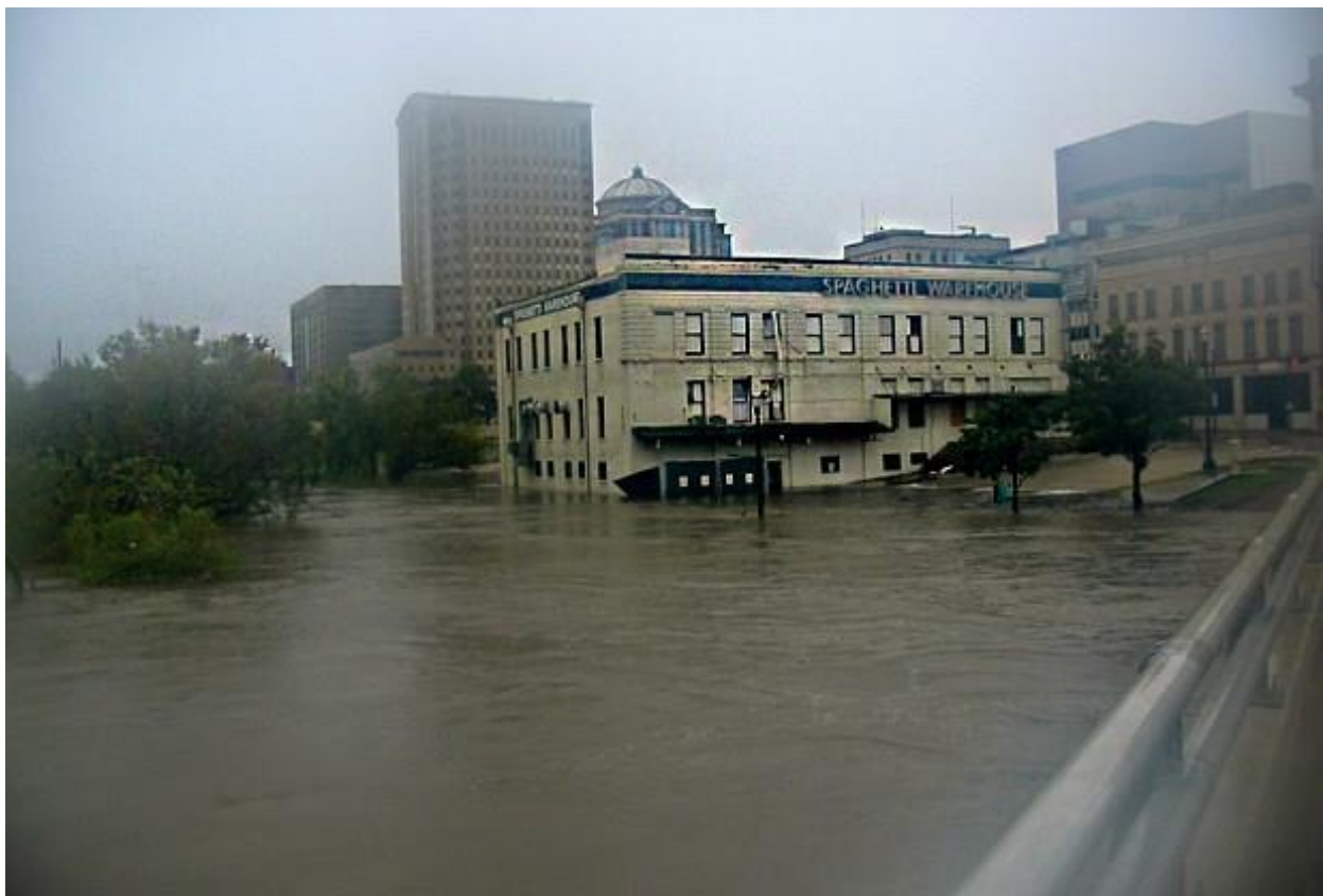
Figure 42. Hurricane Ike- Warehouse in Downtown Houston (2008). Source:(Harris County Flood Control District, 2018)
