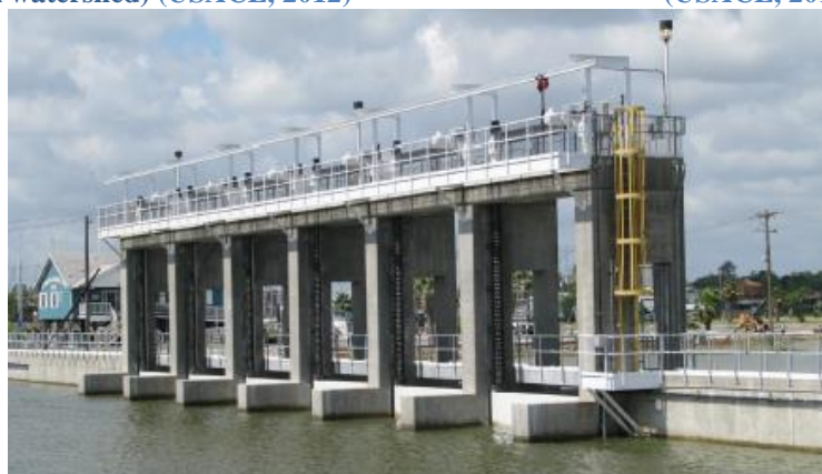
Figure 30. Second Outlet Structure (Gate). Source: (USACE, 2012)
