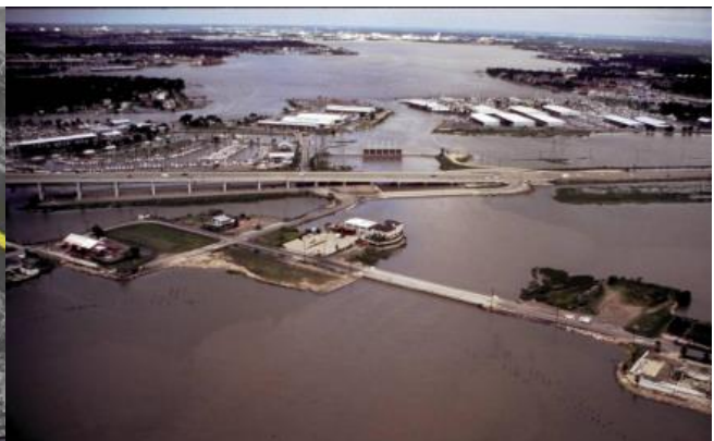
Figure 29. Second outlet channel structure view (USACE, 2012)
