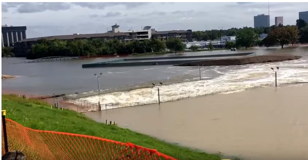
Figure 45. Release of Water through Barker's Dam Spillway - 30/08/2017. Source:(Graham, 2017)
