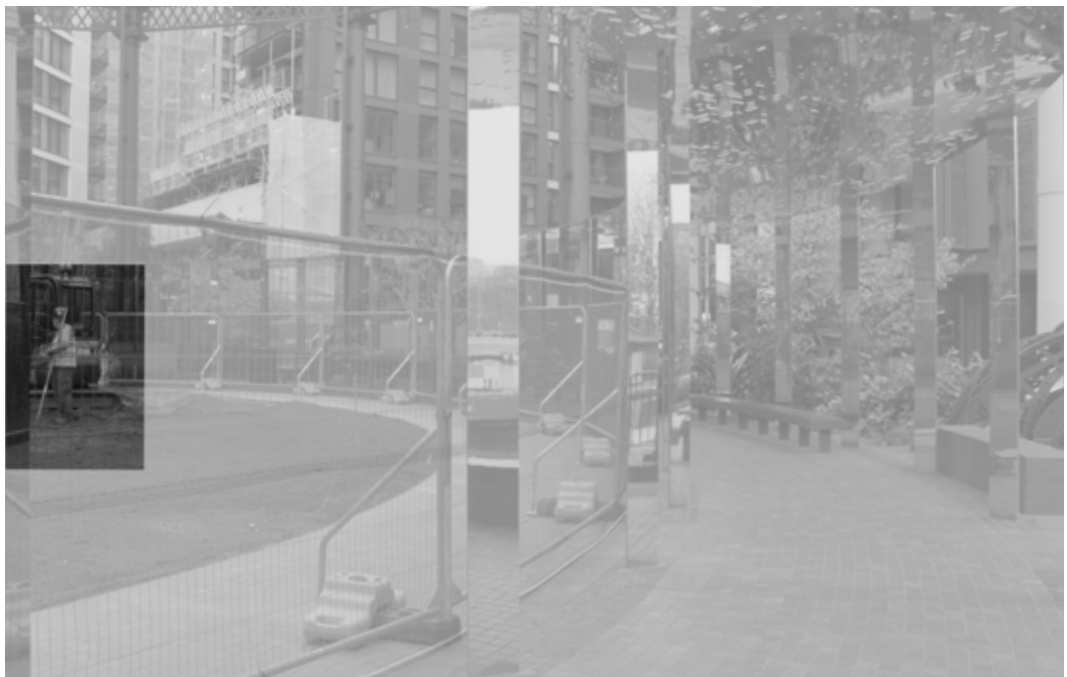
Gasholder Park, under construction Working people Place of traffic and pausing
