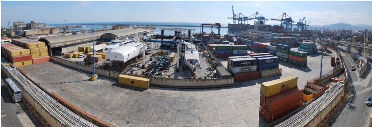
Figure 7 | The Eastern port of Naples. Author's photograph: Paolo De Martino, April 2017.
