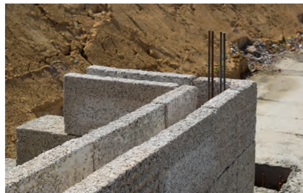
Fig. 50 Installing of concrete hemp blocks Isohemp, 2020 ©2021, IsoHemp - Natural Building
