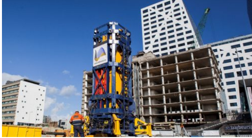
(a) Rapid load test (StatRapid) setup (Allnamics 2021, May 13).
