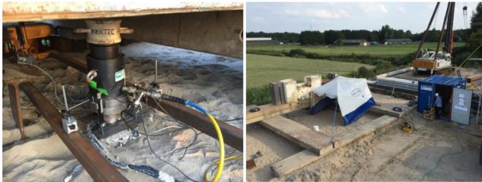
Figure 4.33: Load test setup used at Beemster Tests (NVAF 2019).
