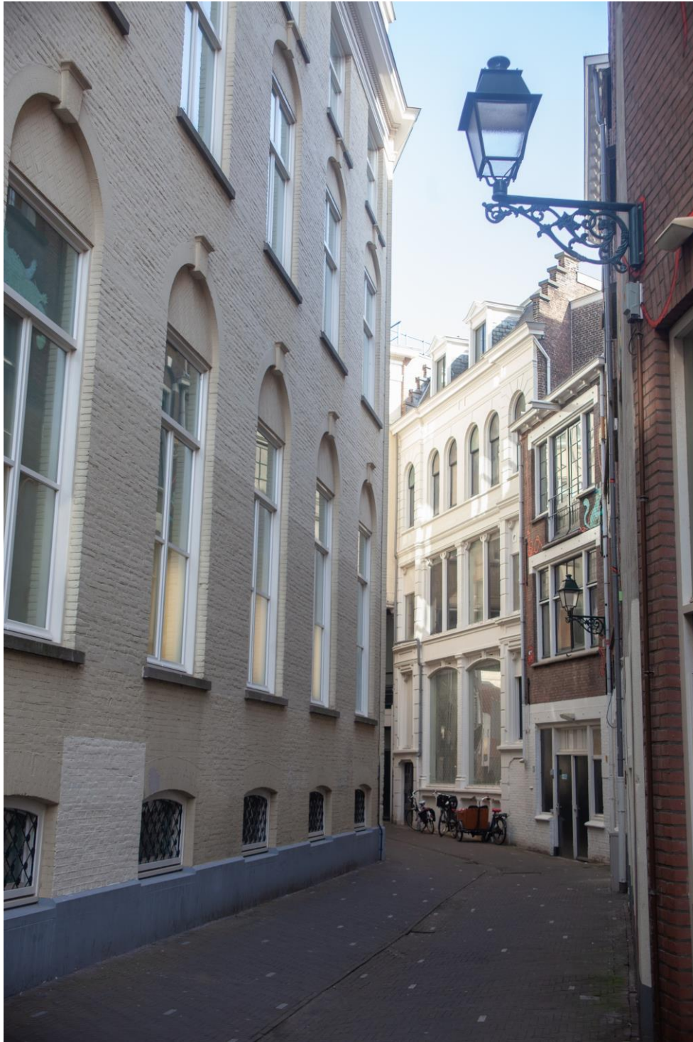
Figure 7 – The back façade of the Passage had to follow the meandering medieval streets of the Achterom
