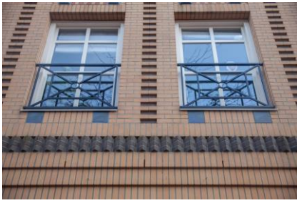
Figure 25 Brick ornament design on The Heuvel's facade
