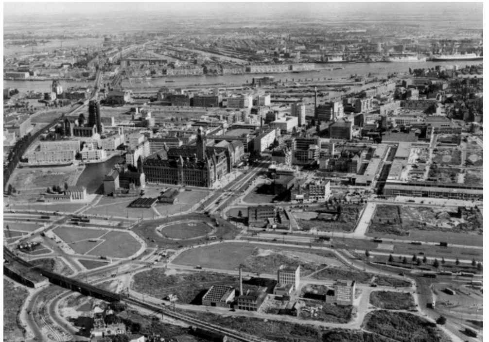
Figure 13 – The Lijnbaan during construction. The difference in scale between the planned roads and the pre-existing city structure can clearly be seen.
