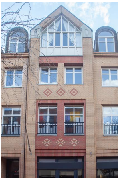
Figure 27 The upper floors are a mix of stock rooms and apartments
