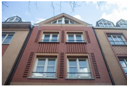
Figure 26 The long façade is disguised as multiple houses with individual roofs
