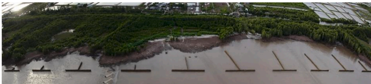
Fig. 15. Placement of T-dams in Bac Lieu Province, Viet Nam (courtesy Cong Ly and G.E. Wind, 2013).
