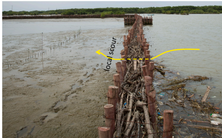
Fig. 29. Example of local scour by near-bed currents underneath loose brushwood, coastal restoration works in Bogorame, Demak, Indonesia.
