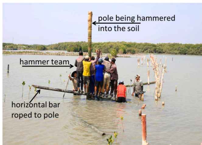
Fig. 32. Hammer team at work to place bamboo pole, Bogorame, Demak, Indonesia.
