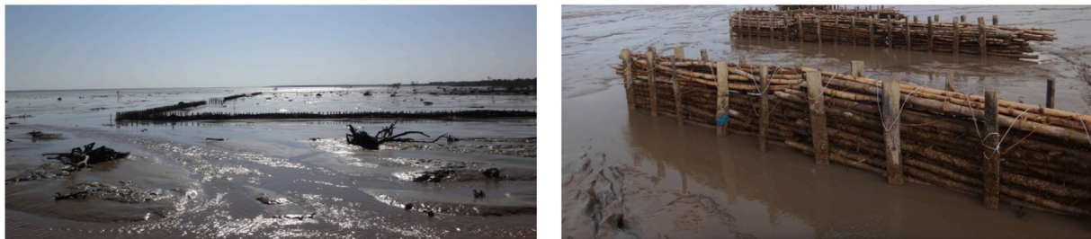
Fig. 11. Permeable dams constructed near Weg naar Zee, north of Paramaribo, Suriname (photos by E. Van Lavieren).
