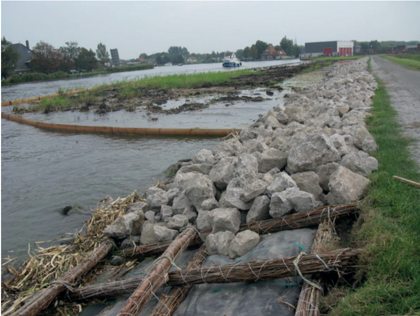
Figure 11-8 Geotextile under mattress (photo Griendhouhandel)
