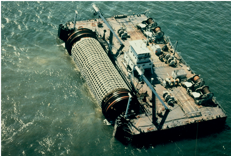
Figure 13-10 Sinking block mat in Eastern Scheldt (Rijkswaterstaat)
