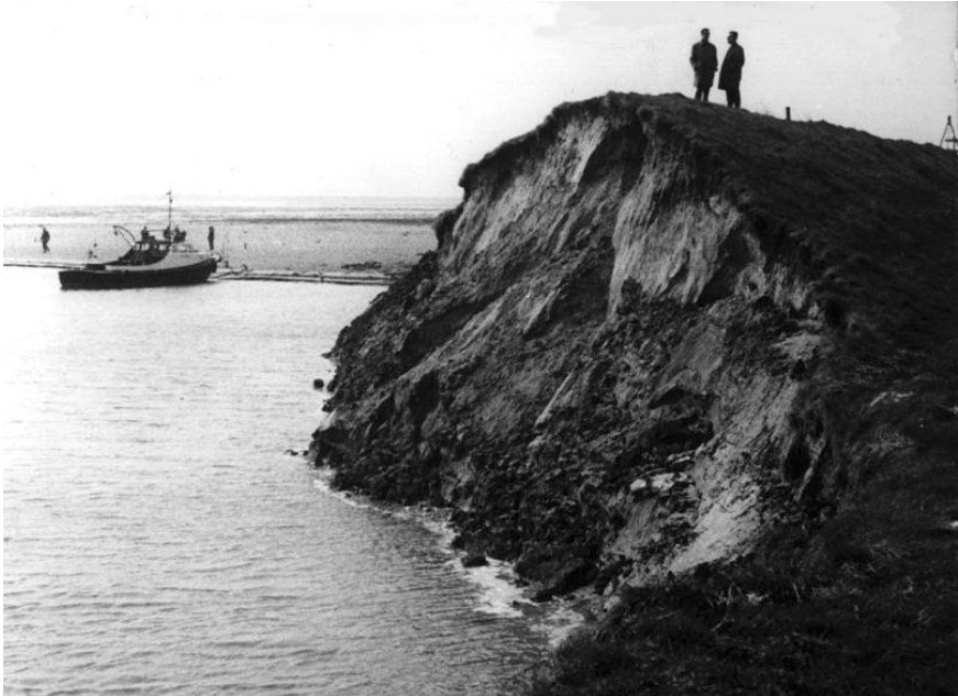
Dike breach ( Dijkval ) in Zeeland, The Netherlands
