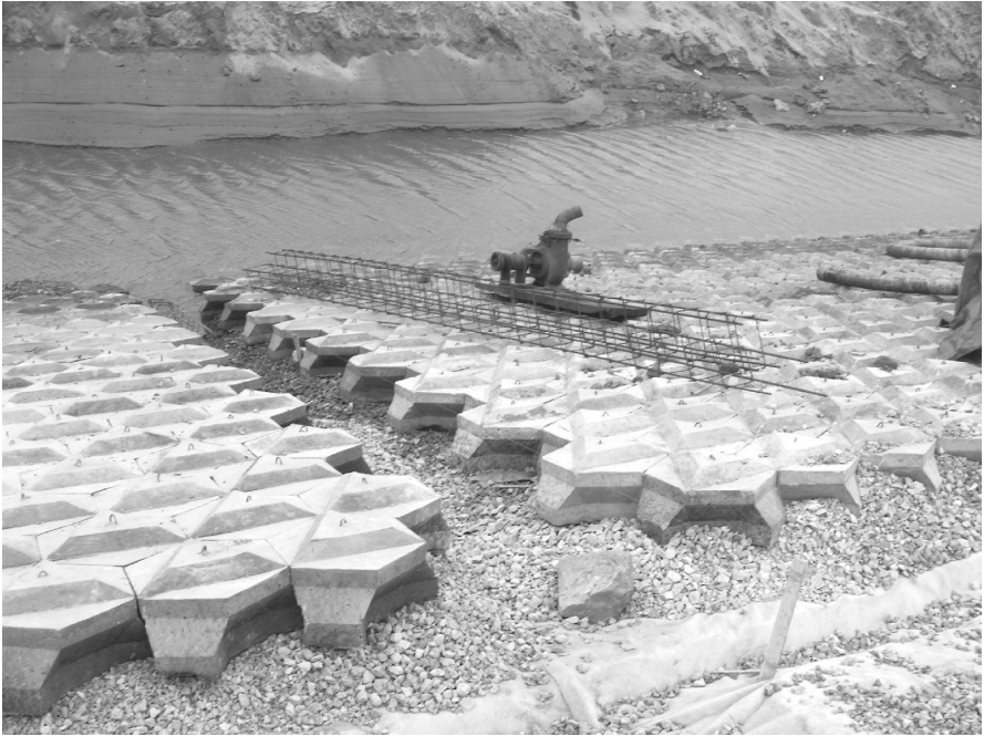
Figure 8-22 Interlock blocks applied in Vietnam (photo Verhagen)
