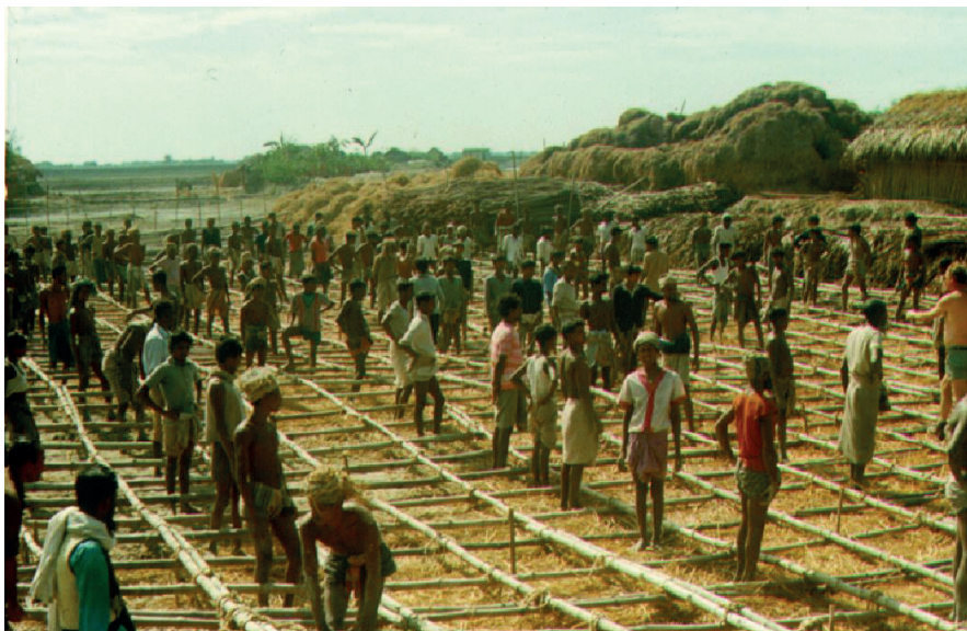
Figure 13-9 Construction of bamboo mattress
