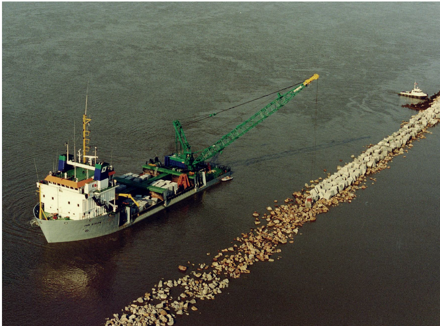
Figure 13-25 Placing elements on a breakwater with crane ship (van Oord)
