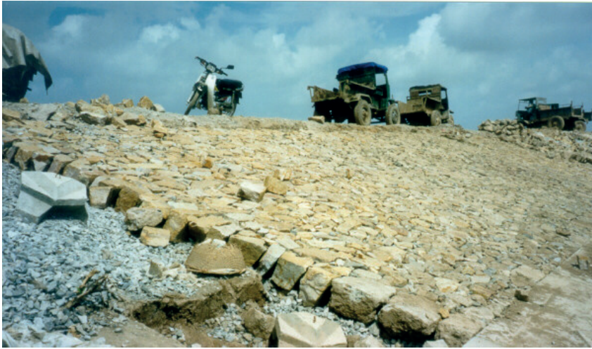
Figure 11-24 Placed block revetment (Vietnam, photo Verhagen)
