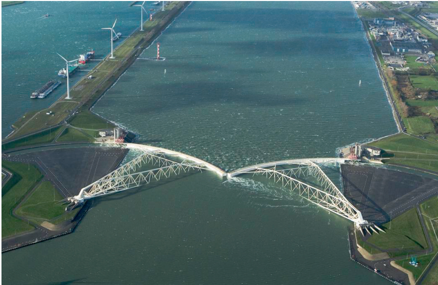
Figure 11-2 Overview Storm surge barrier Rotterdam Waterway (photo Aero Lin)
