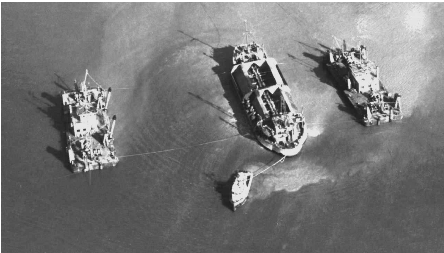
Figure 13-8 Sinking fascine mattress
