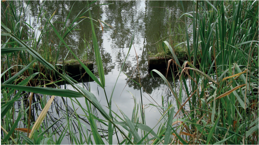
Figure 12-5 Gap in a sheetpile, in this case especially to allow beavers to cross the sheetpile (photo Verhagen)
