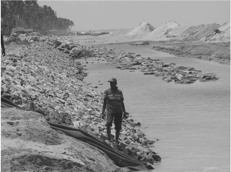
Erosion protection in Sri Lanka (photo Pilarczyk)
