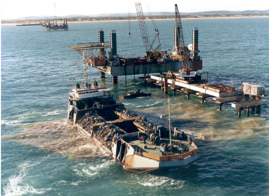
Figure 13-5 Side stone dumping vessel (Boskalis)
