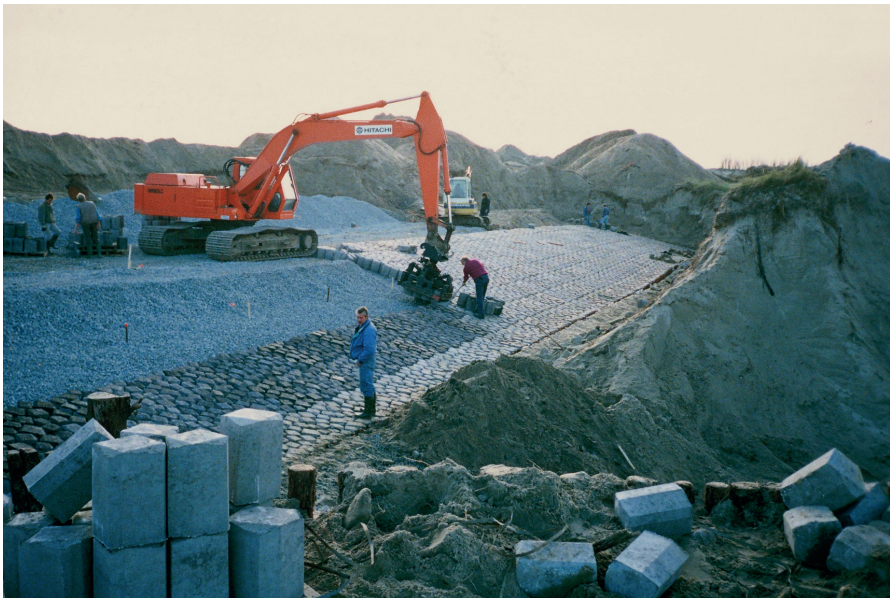
Figure 13-21 Mechanical placement of Basalton (RWS, Hans Johanson)
