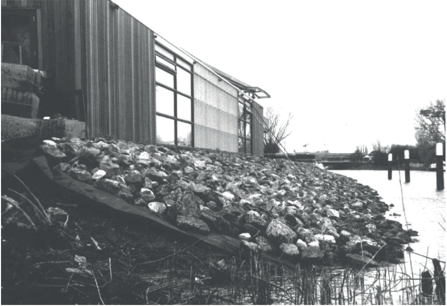
Figure 11-16 Simple bank protection with geotextile
