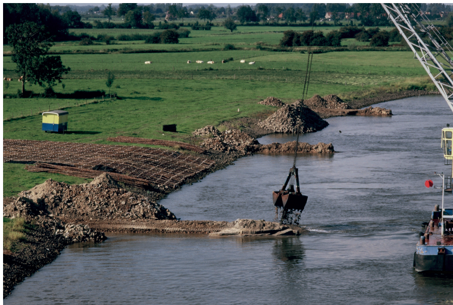
Figure 13-19 Construction of a river groyne (photo Rijkswaterstaat)
