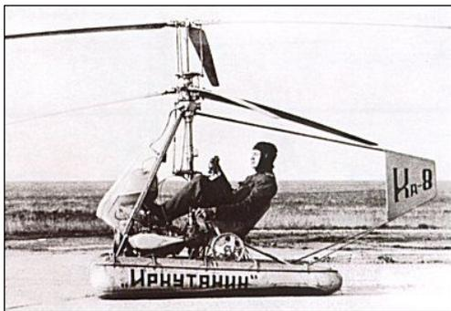
**Figure 3.3:** Kamov A-8 coaxial helicopter (1947). [4]
