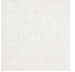
Painted original blockwork
