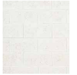
Painted original blockwork
