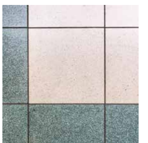
Re-used floor tiles
