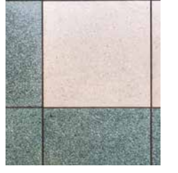
Re-used floor tiles
