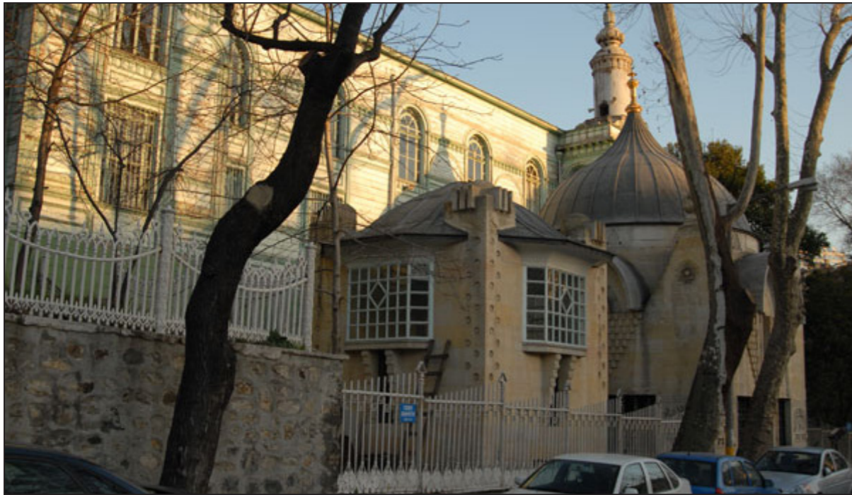
Figure 30: The rough stone fence with... surrounding the mosque
