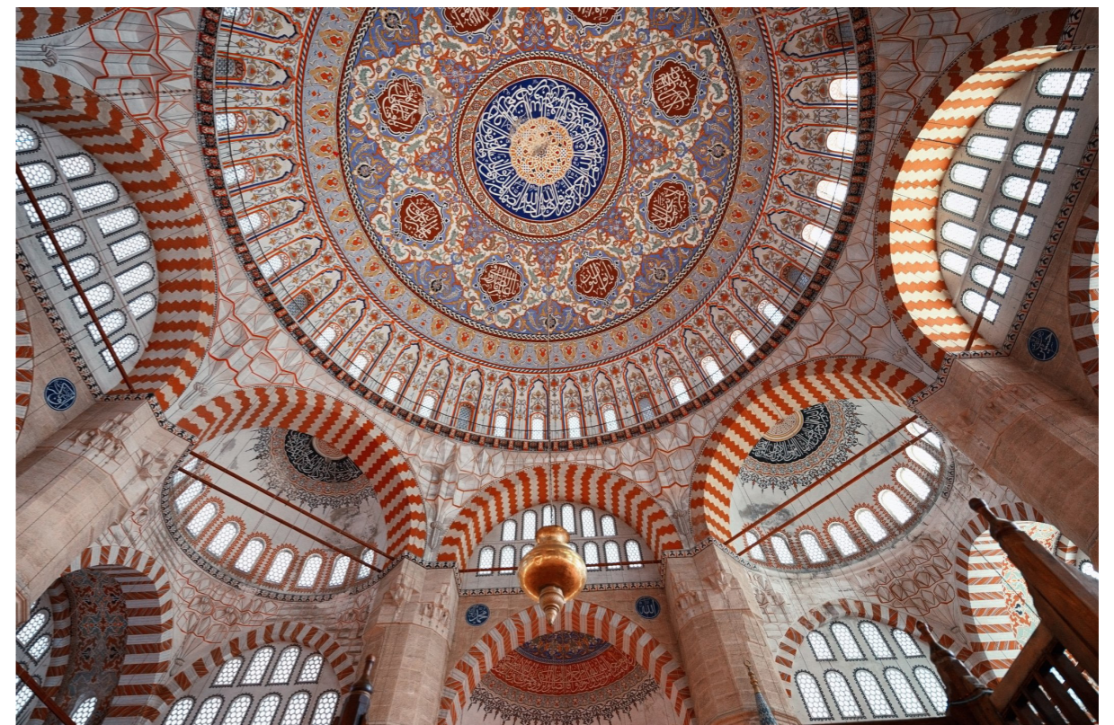
Figure 16: Interior of the prayer hall with the Central “sky dome” and surrounding smaller semidomes
