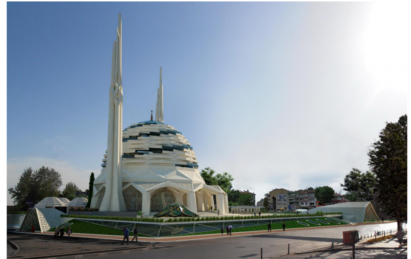
Figure 57: Courtyard of the Mosque
