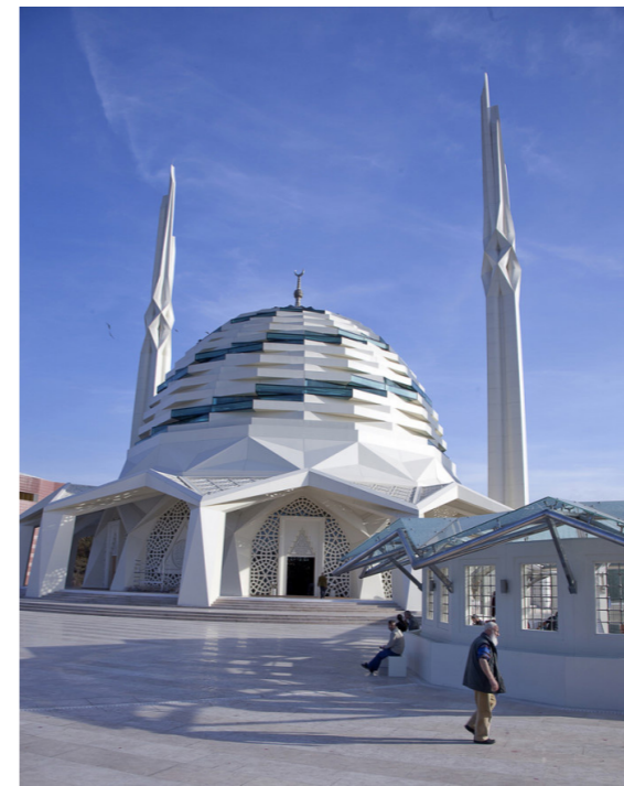
Figure 47: Riwaq in front of the entrance of the mosque
