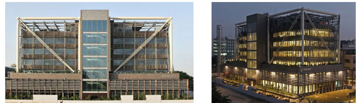
Figure 3.5: Volvo - Eicher Corporate Headquarters (VECH), Gurgaon
