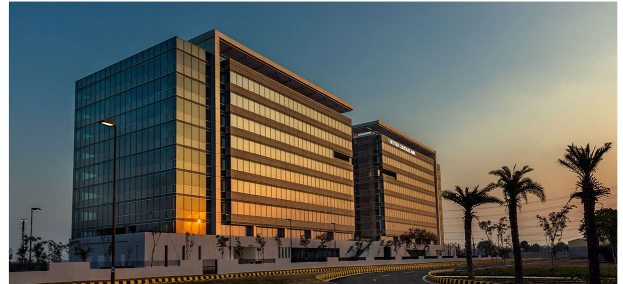
Figure 6.1: Skyview Corporate Park, Gurgaon
