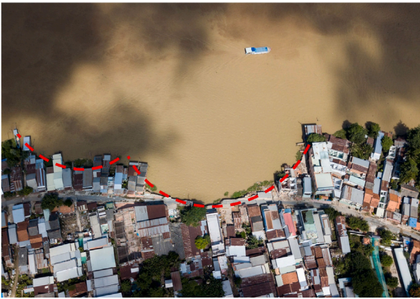
Fig. 3. Bank collapses at Mekong River, Vietnam, due to uncontrolled sand mining resulting in breaching (National Geographic, 2018, photo: Sim Chi Yin). Breaching scars are indicated with red dashed lines.
