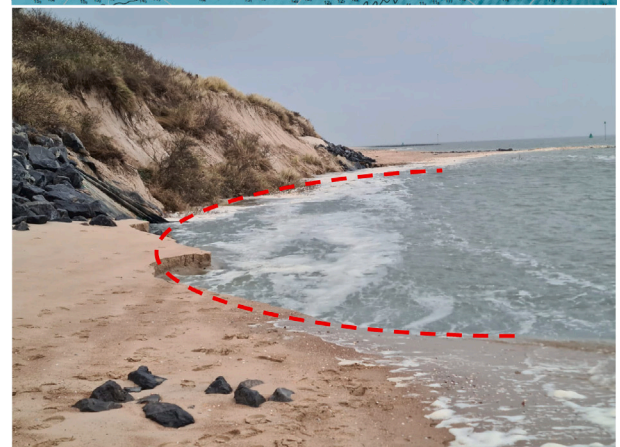
Fig. 10. Beach collapse at Oost-Vlieland between two groynes on January 5th, 2023; post-failure bathymetry (top), photo showing damaged dune foot (Rijkswaterstaat) (bottom). Breaching scar is indicated with the red dashed line.
