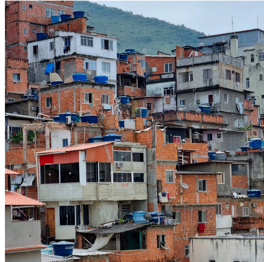
Rooftop water cisterns in Copacabana, Rio de Janeiro (Huub Fenten, 2022)
