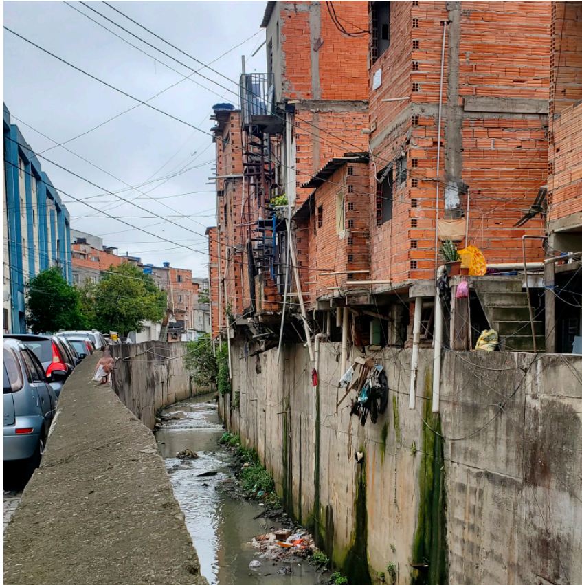
Precarious housing without sewage infrastructure in Heliópolis, São Paulo (Author, 2022)
