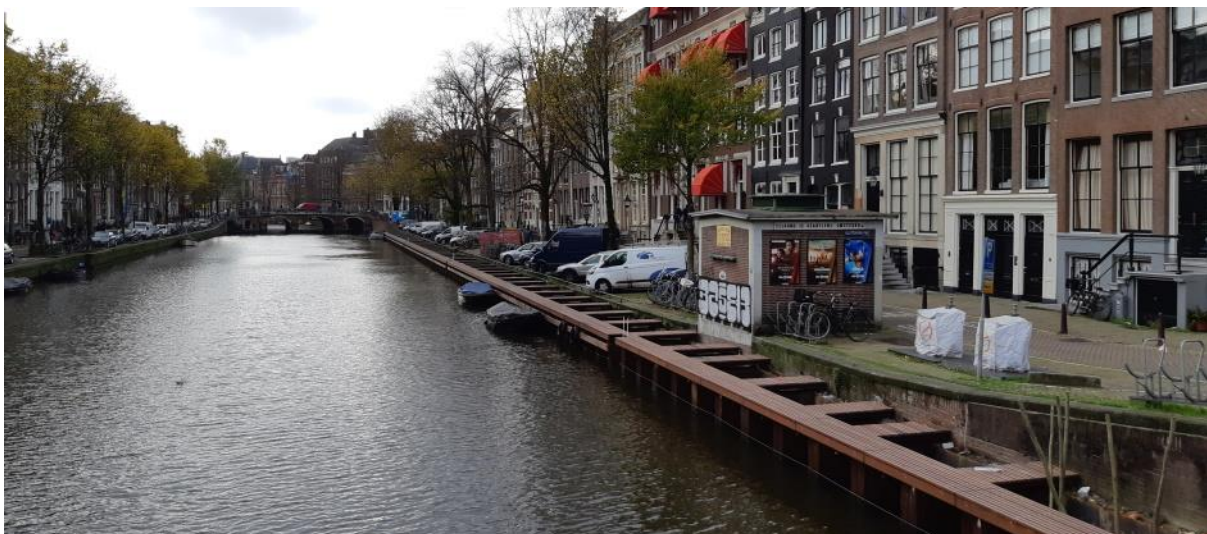
Figure 12. Temporary emergency measurement (Gemeente Amsterdam)
