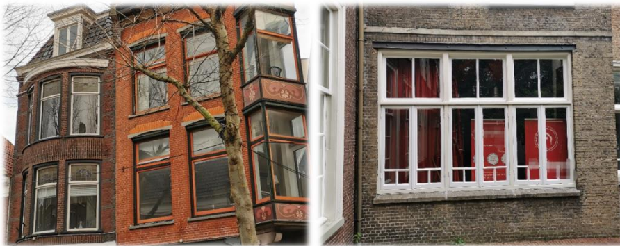
Figure 5.1. Unreinforced masonry walls with large openings in the Netherlands.
