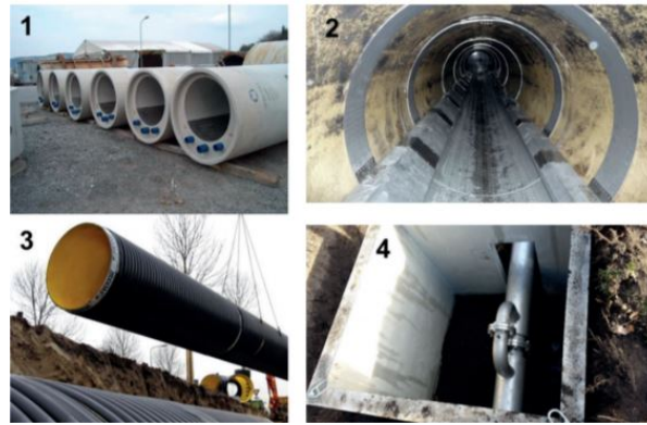
Figure 2.8: Different sewer heat recovery systems. Picture 1 shows a new sewage integrated construction system, picture 2 a standardized sewage build-in system and pictures 3 and 4 a pressure sewage system adaptation (Weeren et al., 2018)
