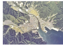
Harbour before complete construction
