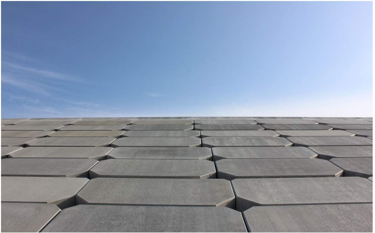
Picture No.12 Huge Concrete walls in Rikuzentakata (Author,2018)
