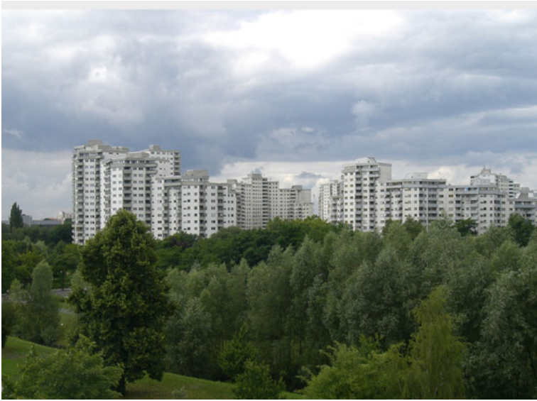
Fig. 5.3 Märkisches Viertel: residential towers on Senftenberger Ring by Chen-Kuen Lee (left and right in foreground) and by Heinz Schudnagies (middle in the background), built 1964. Source Florian Urban 2009
