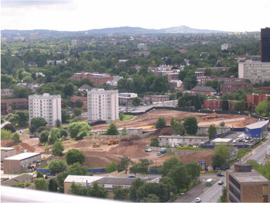
Fig. 6.9 Refurbished tower blocks alongside cleared sites being prepared for new parks and new mixed-tenure housing. Source Birmingham Library Archives and Optima Community Association, used with permission
