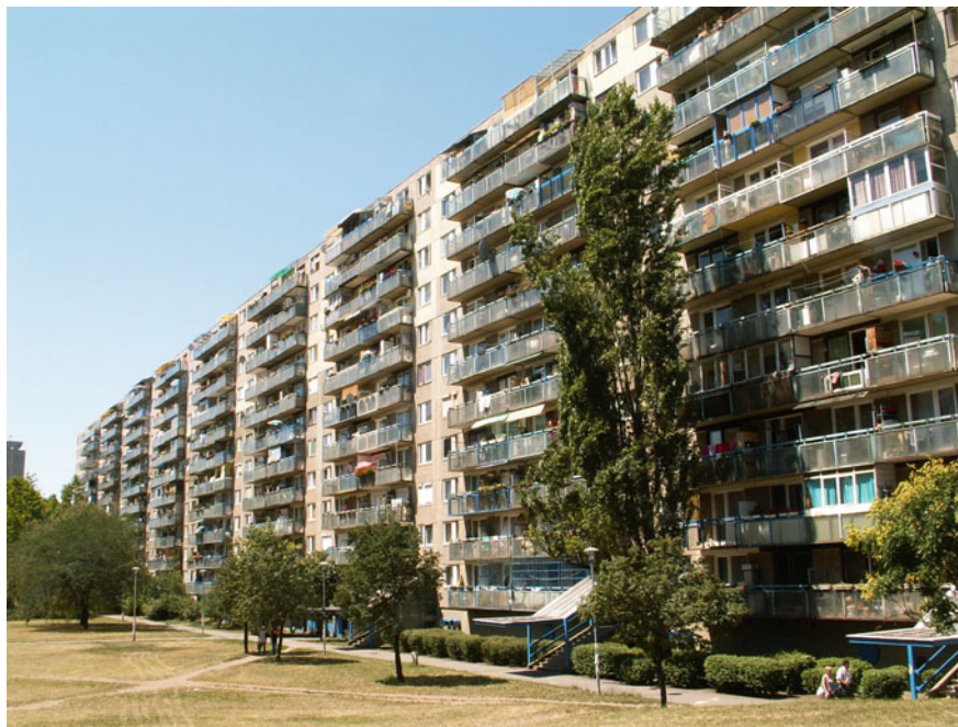
Fig. 9.5 Havana housing estate in the 18th district of Budapest, built using pre-fab technology in the late 1970s. Source Kovács, Egedy and Szabó
