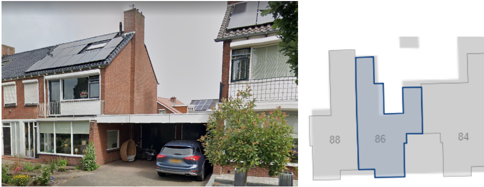
Figure 6.3: Google street view of building ‘NL.IMBAG.Pand.1742100000008886’ (left) and its footprint (right).
