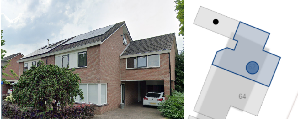
Figure 6.1: Google street view of building ‘NL.IMBAG.Pand.1742100000007039’ (left) and its footprint (right).
