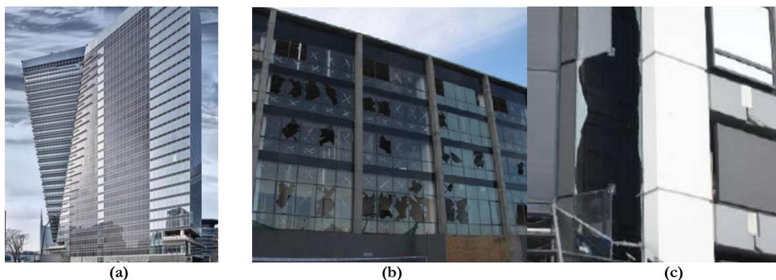
**Figure 1. (a) Application of unitized curtain walls to high-rise buildings - GIOIA 22 tower in Milan, Italy (by Permasteelisa S.p.A.). Seismic damage to glazed facades: (b) 2010 Chile earthquake [FEMA E-74, 2011], (c) 2011 Christchurch earthquake [Baird *et al.*, 2011]**
