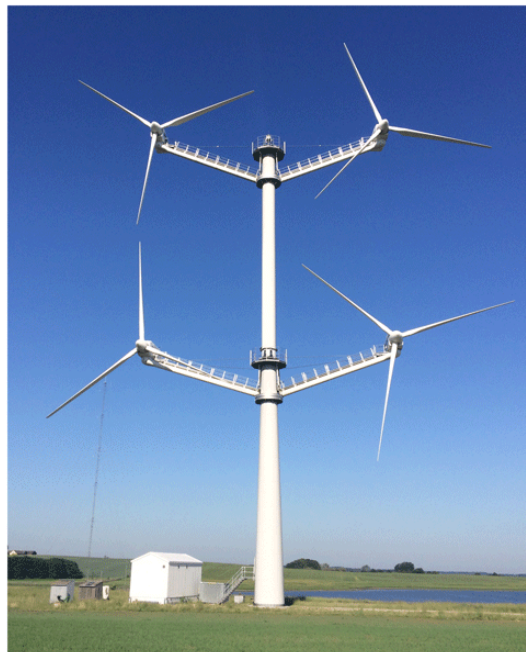
Figure 1.1: Vestas 4R-V29 multi-rotor wind turbine [van der Laan et al., 2019].
