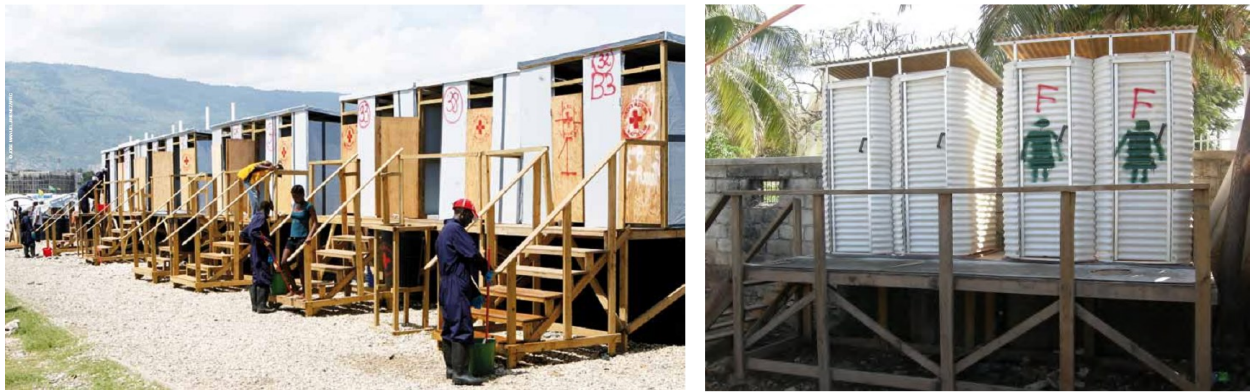
Figure 2-7. Raised toilet units in Haiti (Oxfam, 2011b)
