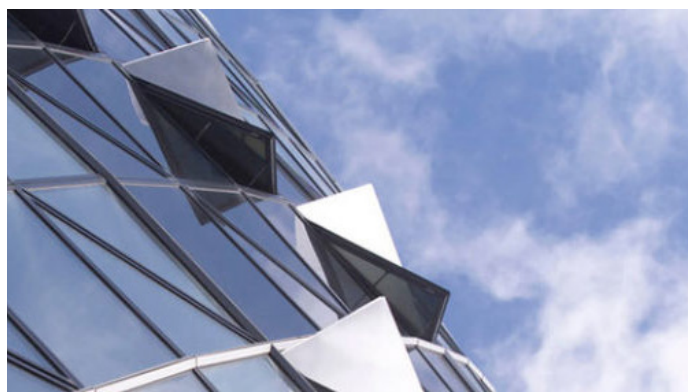
Fig. 2.13. The left and top right image depict the highlight towers and its natural ventilation system, source: http://www.rumausbau.apleona.com/en/apleona-rm-usbau/references/high-rises/highlight-towers-munich/ , Fig 2.14. The picture indicates the openings in atria of 30 st. Mary axe, source: https://www.archute.com/the-gherkin-a-monumental-building-in-the-middle-of-london-by-foster-partners/img13/
