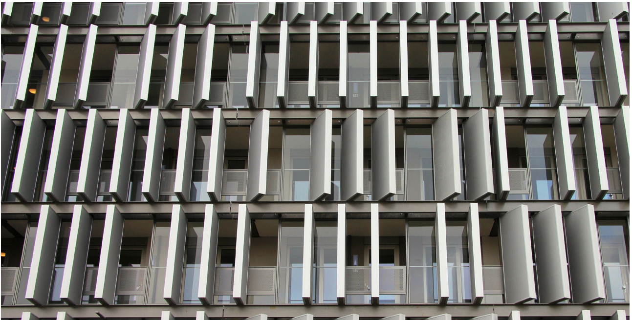
Fig. 2.11. The image indicated Laan van Spartaan facade where coulissen are applied to reduce noise exposure, source: http://weekblad.cobouw.nl/digitaaleeditie/2012/2/20120316___/1_08/article11.html
