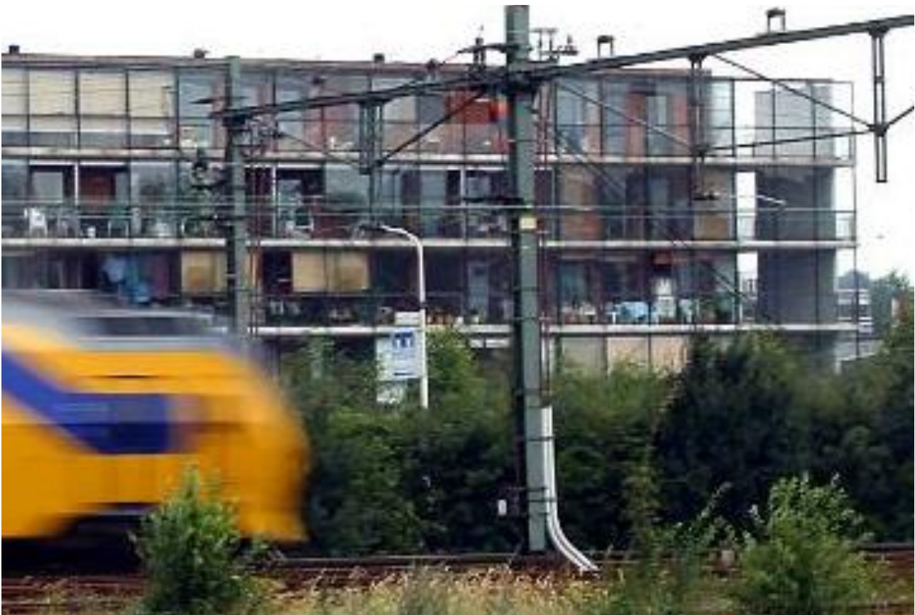
Fig. 2.8. Double skin facade installed in residences in Delft as sound barrier, source: Building Physics lecture acoustics 1 AR1B025
