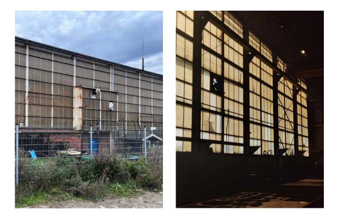
Using the same proportions and facade repetition as the original shipyard. Using simple but smart curtain wall technique to achieve slim steel profiles with single translucent glass panes.
