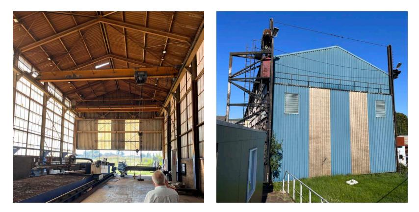
The full facade door and counterweight structure are transferred to the new shipyard, where it will be fully functional. Reinforcing the connection with the waterfront, which was lost when the new dike was build.
