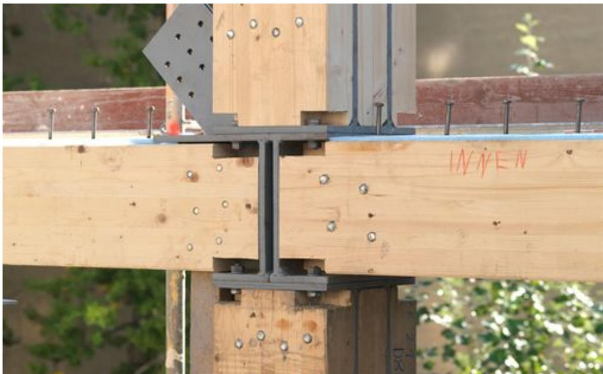
Figure 2.14: Additional steel components applied to transfer the normal forces from one column to the other
