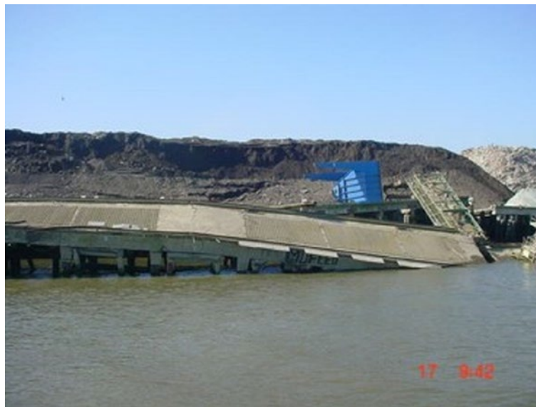
Figure 5. Failed jetty.
