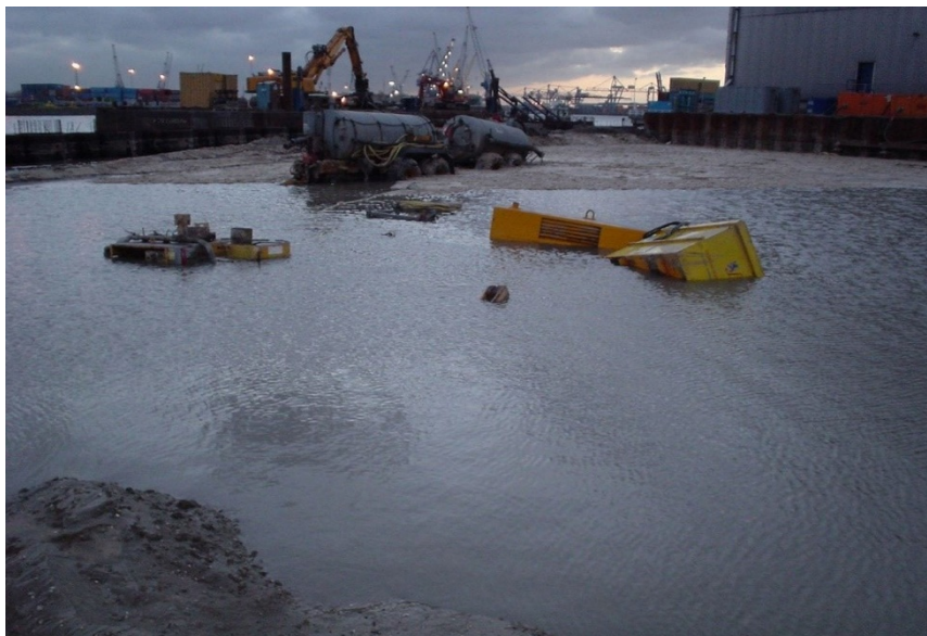
Figure 12. Flooded excavation.
