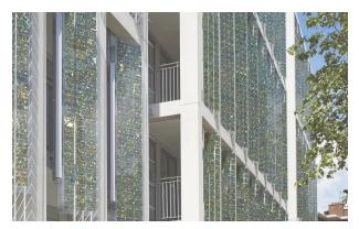
Figure 117: Vertical louvres with integrated PVs. The PVs are given shades of green and gold in order to integrate with the environment and appear as a 'living wall'.
