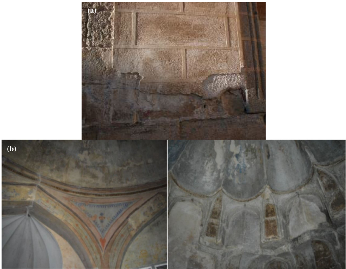
Fig. 3 a Durability of air lime render imitating stone over stone masonry in Évora Cathedral, in Portugal (seventeenth century); b Interior of Pasa Hamam, Thessaloniki (1530 AD), with well-
