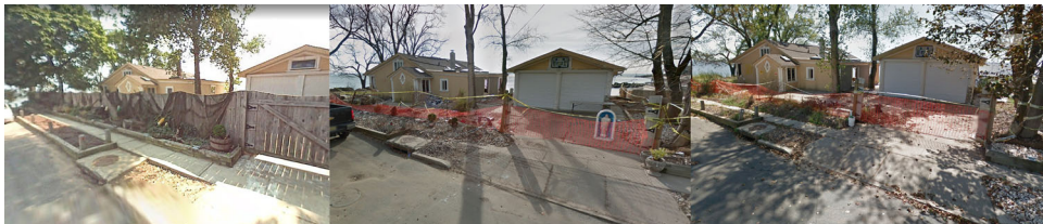
Figure 9. Comparison of one of the buildings in the study area utilising Google Street View, from left to right: September 2007, January 2013, September 2013. The far left image is prior to Hurricane Sandy, while the middle image is 2–3 months after the hurricane and shows extensive damage to the sidewalk and fence. The image on the right is roughly a year after the hurricane and the damage to the fence was still present. Source: Google, 2018.
