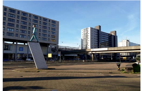
Pedestrian bridge on the North side of the station
