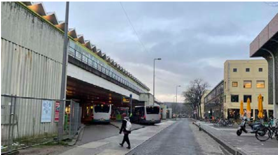
The station counts with an elevated metro line and bus services at ground level. This area is targeted for renovation enhancing passenger experience.
