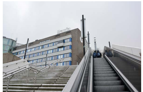
Stairway to pedestrian bridge on South-East side
