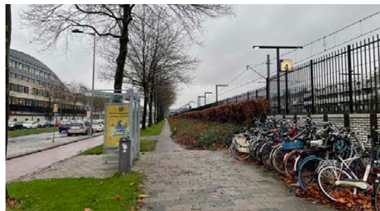
The train tracks establish an access barrier dividing the Feijenoord borough and the Kop-van-Zuid - Entrepot borough. Car and train traffic also cause noise nuisance
