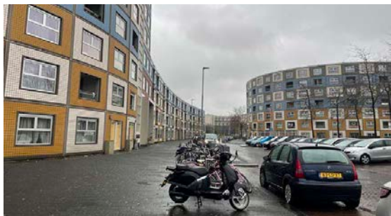
The area is characterized by the presence of social housing, including the remarkable Paperclip. Although in proximity to the train station, this area has a relatively small population in comparison with the other 8 boroughs of the Feijenoord District.
