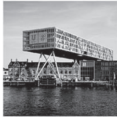
2019 Upfield The Attic
