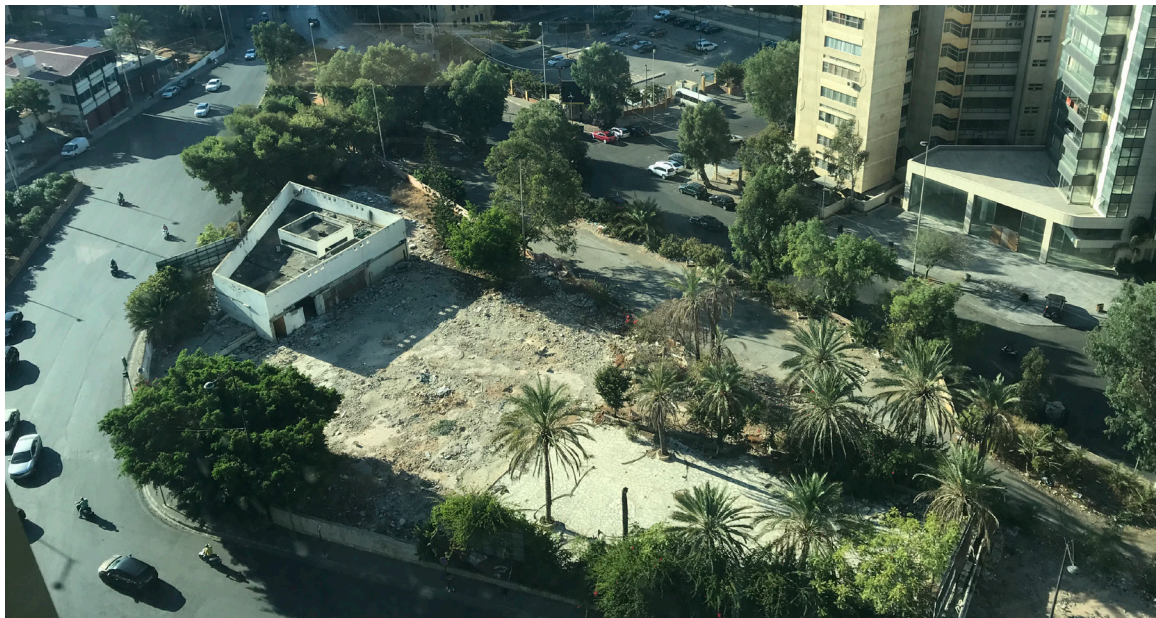
Fig. 5: Aerial of the project location (own picture)
