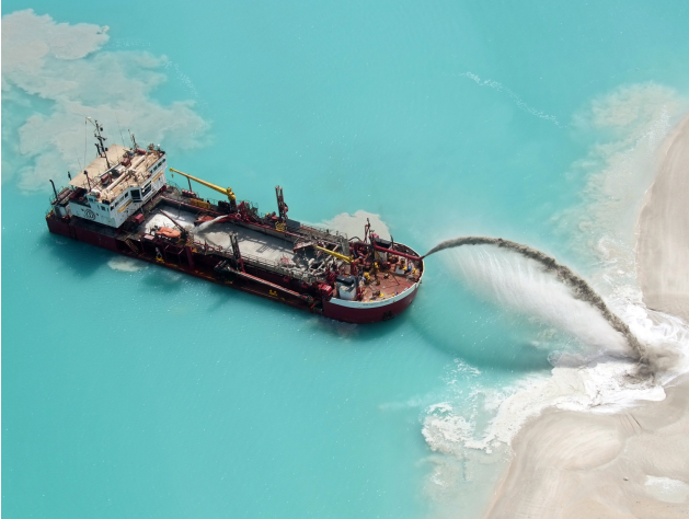
Figure 2.1: The TSHD Northerly Island rainbowing (Original from: GLDD)
