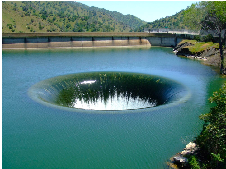
Figure D.12: Morning glory spillway
