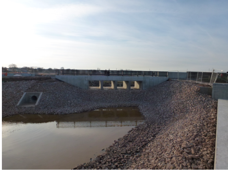
Figure D.11: Culvert spillway type
