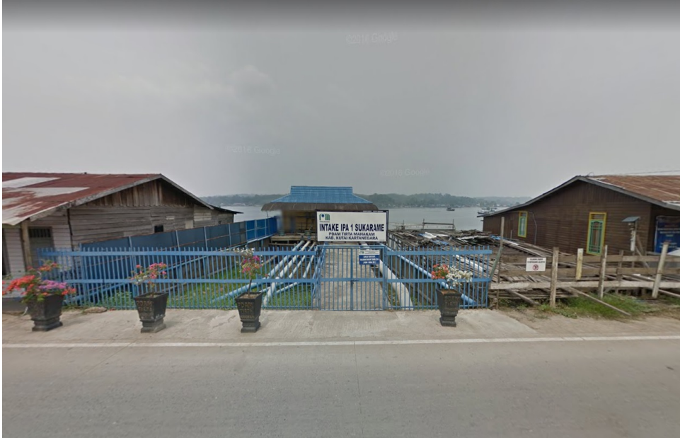
Figure E.4: PDAM Tenggarong Mahakam River pumping station ( Google Earth )
