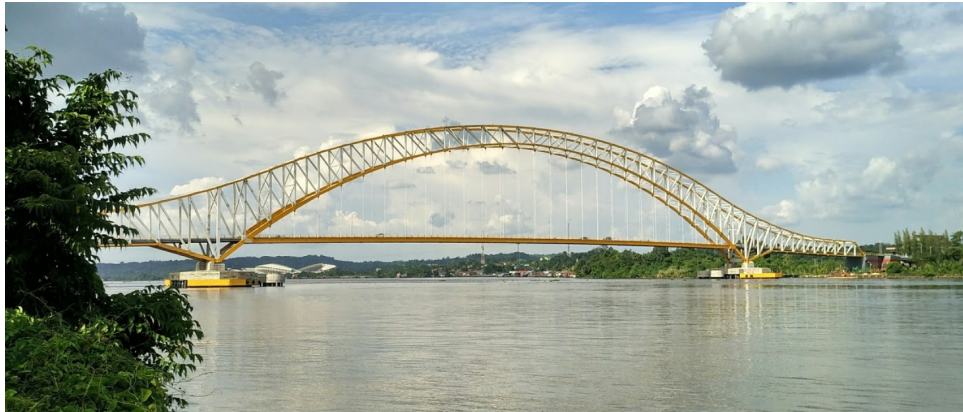
Figure E.8: Kartanegara Bridge
