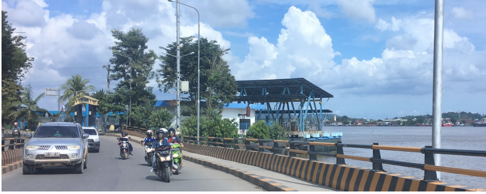
Figure E.2: PDAM Mahakam River pumping station (own work)
