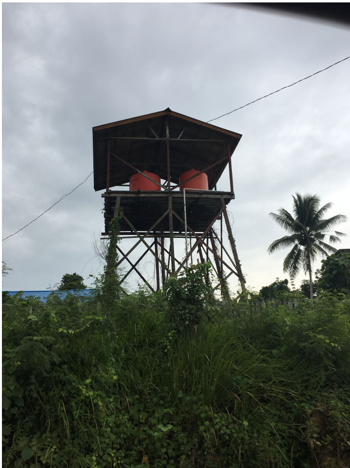
Figure E.9: Water tower in Kenangan, Indonesia ( Own work )
