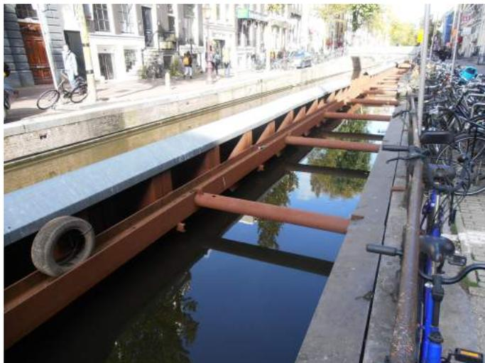
Figure 5.21: Temporary sheet pile construction at the Oudezijds Achterburgwal
