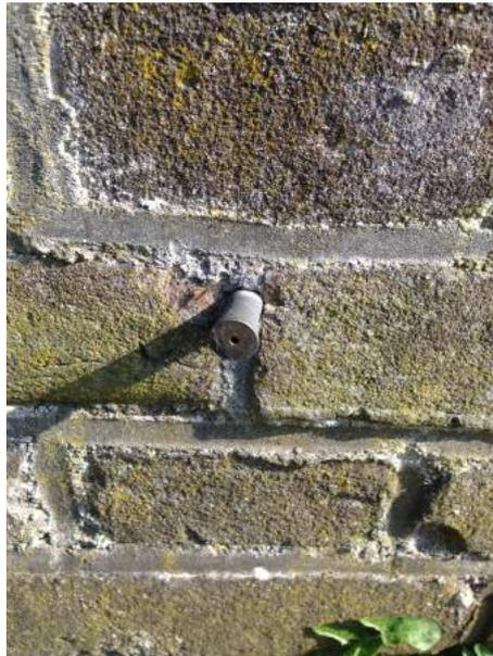
Figure 3.1: levelling benchmarks on a building of the Spoorsingel in Delft
