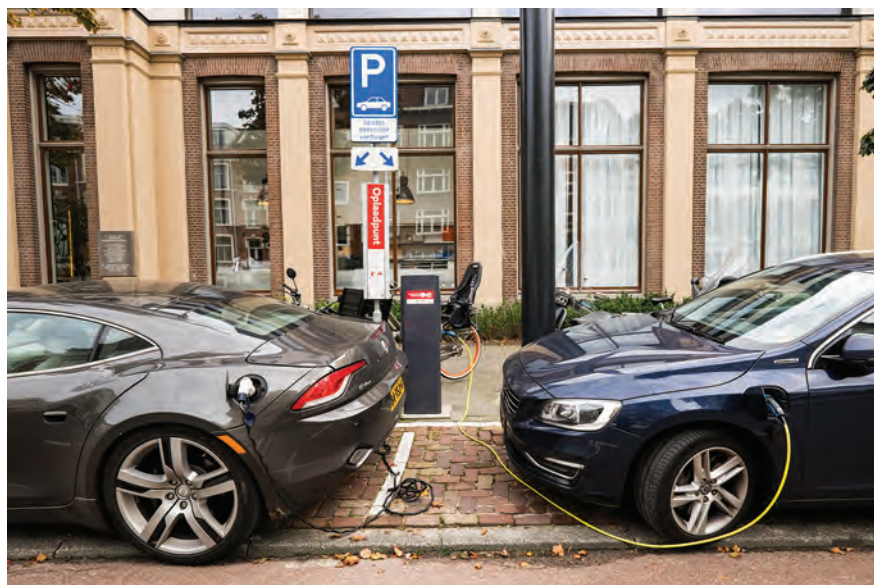
Figure 1.1 Electric cars at a public charging station in Amsterdam. (Photo: Michiel Wijnbergh)
