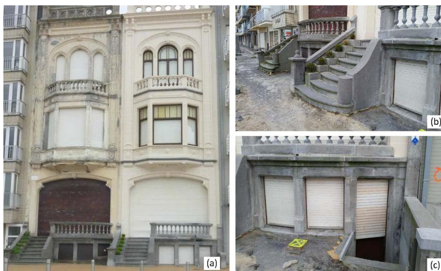
Figure 10. Typical old apartment buildings on the Belgian coastal dikes. (a) Front view of apartment buildings (built in 1913); (b) stairs to the ground floor; (c) entrances of the basements closing by shutters.
